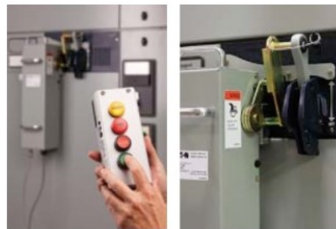
Ampgard remote operator
